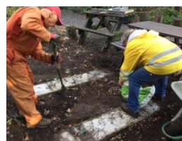
Putting in concrete blocks
