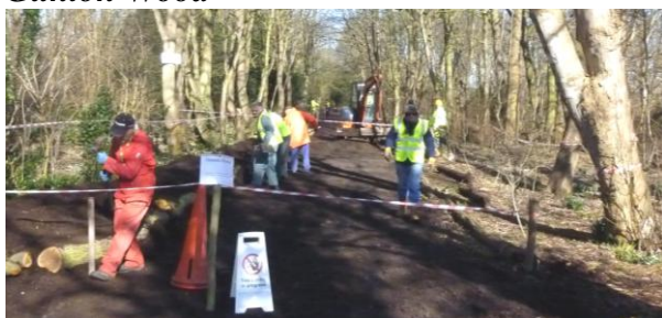
Working on the main footpath
